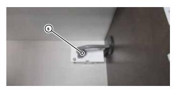
5. Remove the six screws <sup>1</sup> holding the microwave in place.
