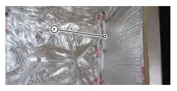
8. Remove the access panel <sup>®</sup> by removing the staples first.
