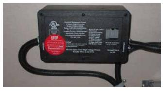
When shore power is connected it passes through the EMS-LCHW30 surge protection device to protect the wiring in the Unity.
